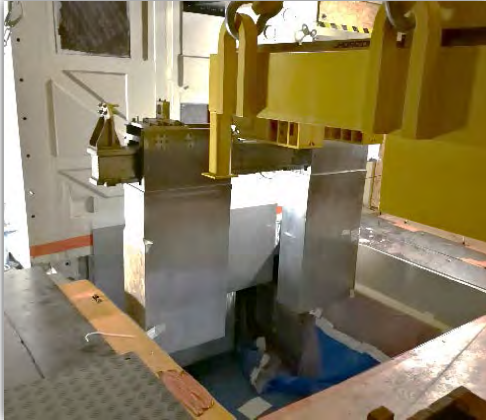
installation with use of EMZ crane
